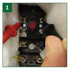
No Hot Water Check for power at top two screws of upper thermostat. If 240V not present, check circuit breaker/wiring.
