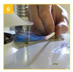
Thermal Switch Tripped (Air Supply Problem) If the thermal switch tripped, it is likely an air supply problem. Clean air filter and flame arrestor. Room must supply adequate air. Conduct "draft test." Turn main burner on. After five minutes of main burner operation, smoke source should be drawn into draft hood. If not, you have an air supply/venting problem.
