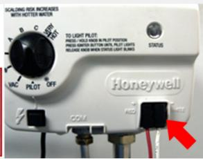
Make sure the black connectors are firmly attached to the gas control valve.
