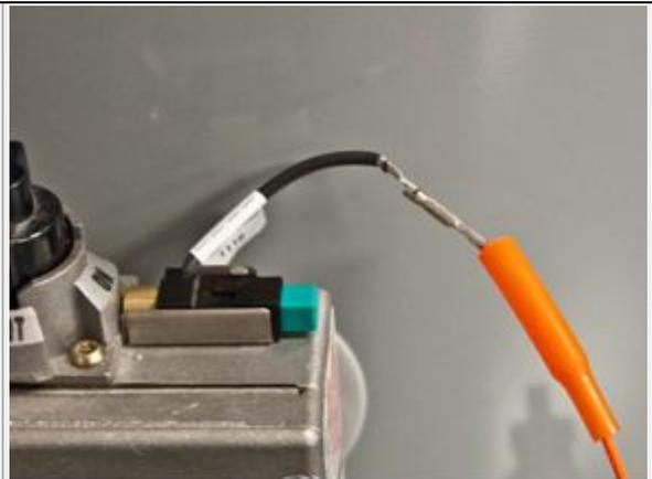
The black and orange igniter wire connectors must be firmly attached together.
