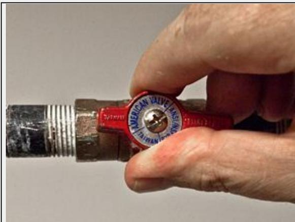
Make sure the manual gas supply valve is ON.
