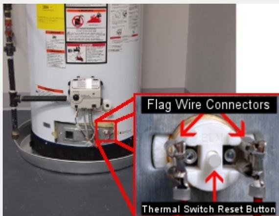
Make sure the two thermal switch wires are undamaged and the wire connectors are firmly attached to the thermal switch.
