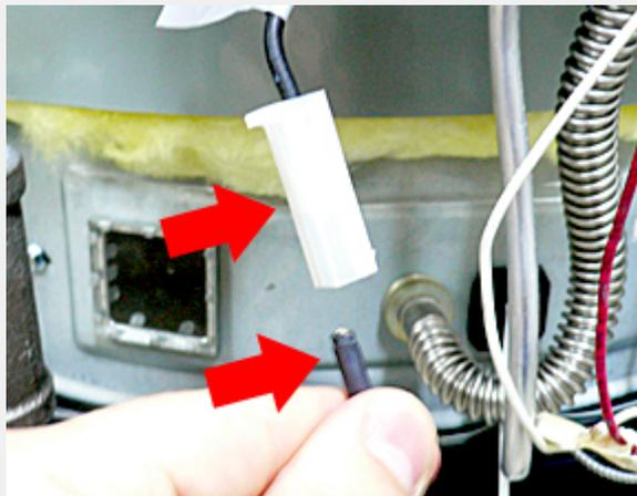
The igniter wire must be firmly inserted into the white connector.
