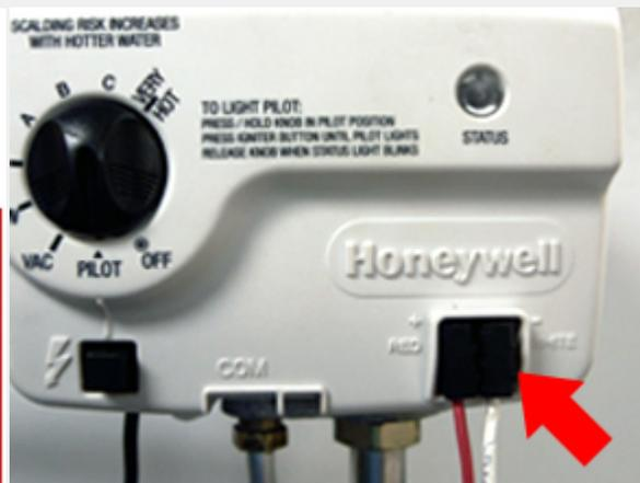
Make sure the black connectors are firmly attached to the gas control valve.
