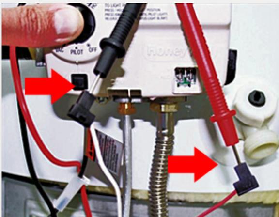
Use a multimeter to test the millivolt output of the thermopile.
