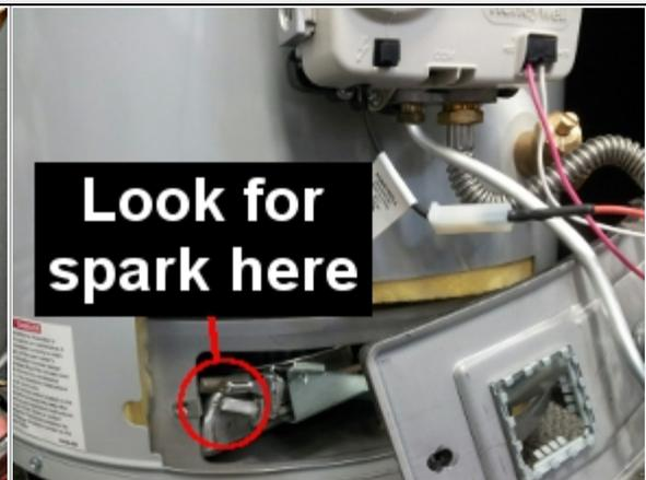
If you can't see a spark through the viewport, pull out the burner assembly and check for a spark near the igniter.
