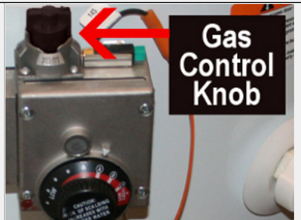
Gas control knob location on gas control valve.
