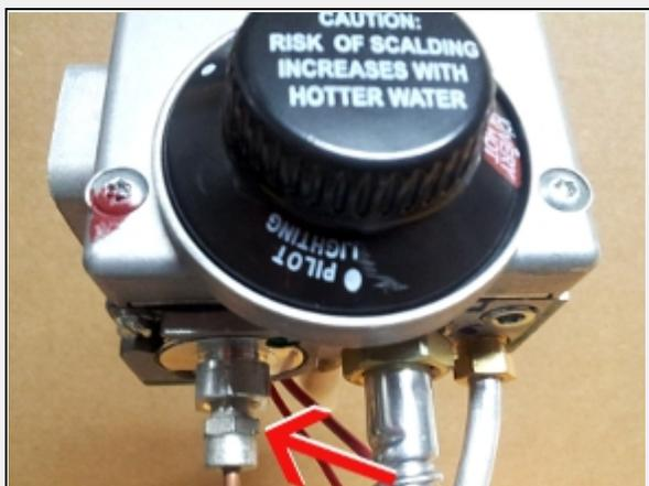
**Check/tighten the thermocouple connection.**
