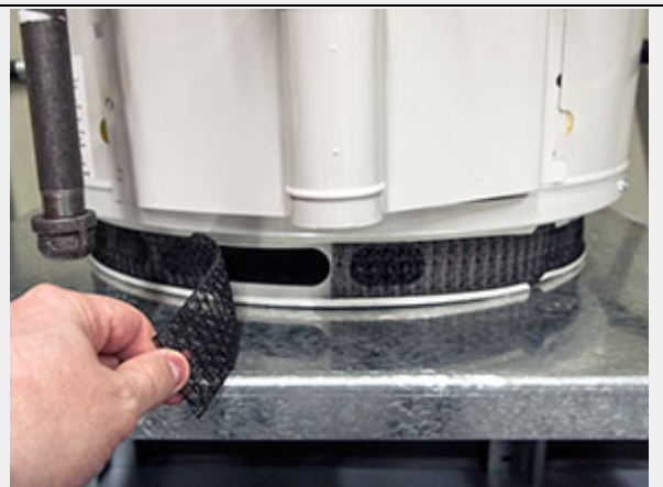
This model has a long, slide-in filter screen that wraps around the entire base of the unit).
