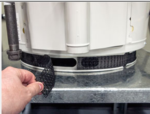
This model has a long, slide-in filter screen that wraps around the entire base of the unit).
