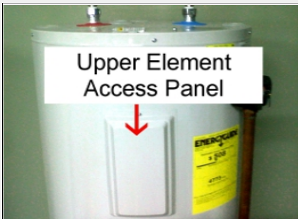
Upper Element/Thermostat Access Panel.
